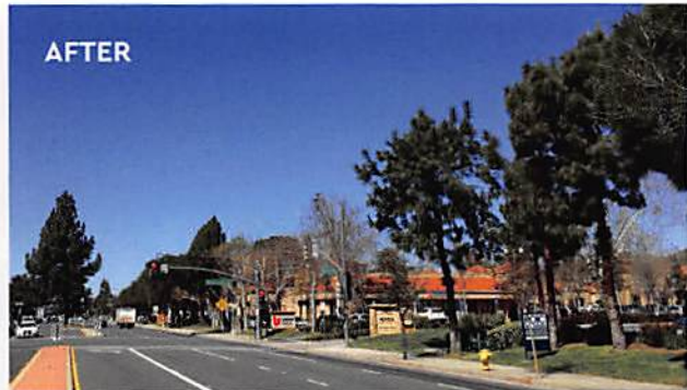
Thousand Oaks Blvd. Undergrounding
